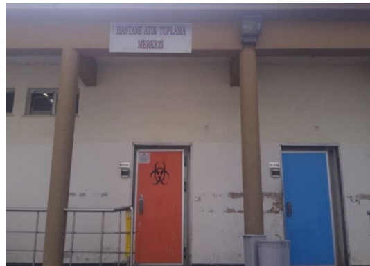
Faculty of Medicine Waste Temporary Storage Area
